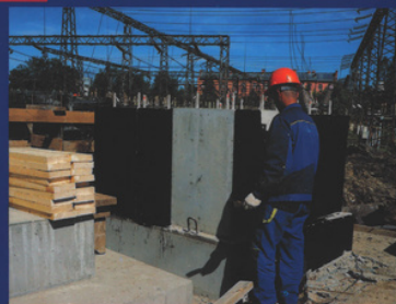
CONCRETE & BLOCK FOUNDATION WATERPROOFING
