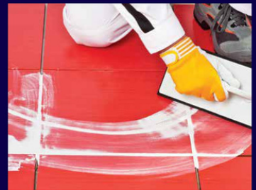
APPLYING TILE GROUT
