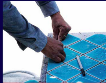
FIXING TILES ON POOL STEPS
