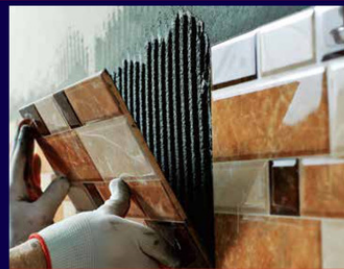
FIXING CERAMIC TILES
