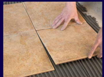
GLUING TILES
