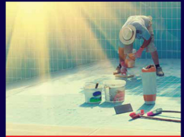
FIXING SWIMMING POOL TILES
